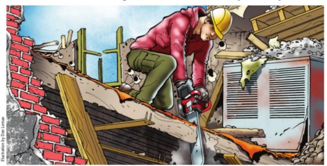
The accident: A construction company was demolishing a twostory warehouse. A large portion of the building had already been razed when the second floor collapsed onto the first, trapping three workers. Emergency personnel worked to support the hole to keep it from collapsing further while attempting to rescue the workers. One worker was killed and two others were injured.
