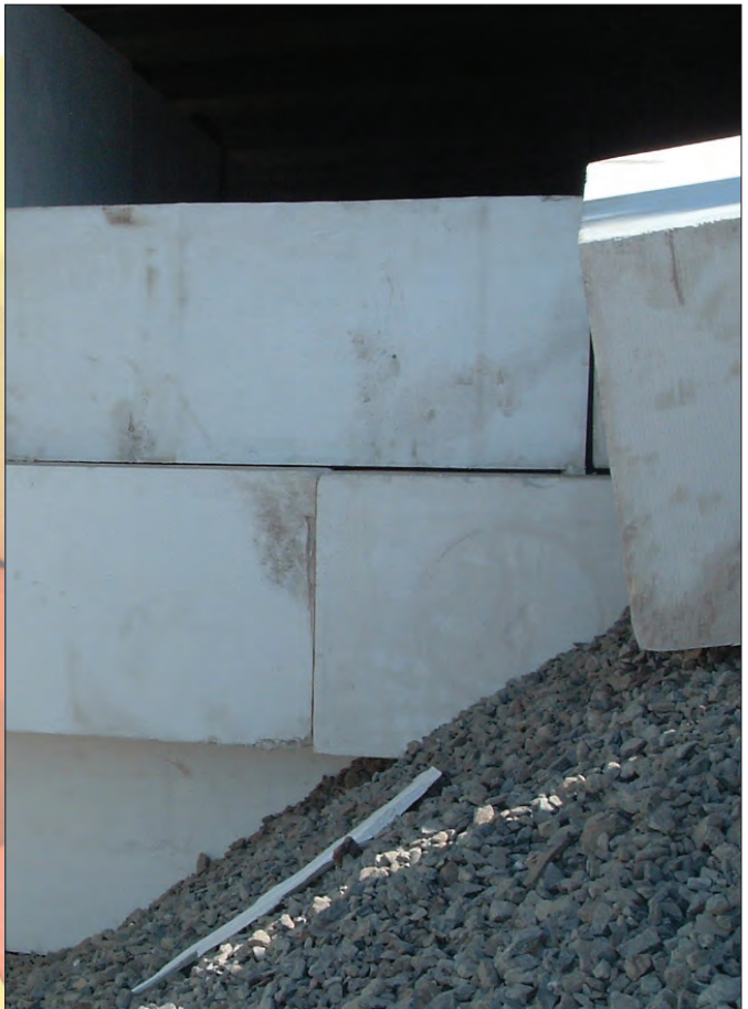
Geofoam blocks were stacked behind the abutment wall as backfill on the I-215 at 3300 South bridge project.
