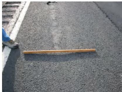
Figure 2.18: Rutting on I-90 in Washington State attributed to stripping of the underlying layer
