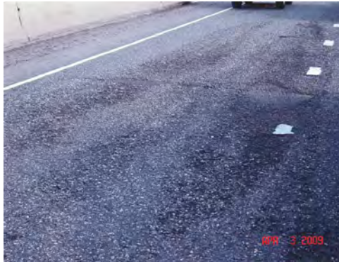
Figure 2.14: Delamination following raveling on I-5 MP 307.60 SB in Oregon.
