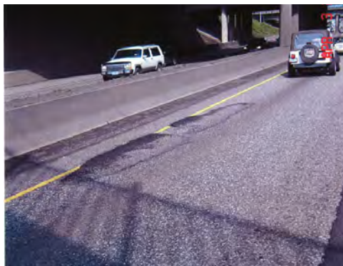
Figure 2.16: Patched delamination on I-5 MP 302.30 SB in Oregon
