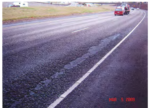
Figure 2.17: Delamination following raveling on I-2055 MP13.74-15.98 in Oregon following winter 2009 snow storms
