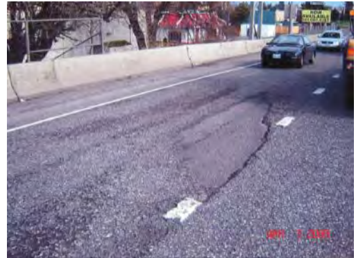
Figure 2.15: Delamination following raveling on I-5 MP 307.70 SB in Oregon
