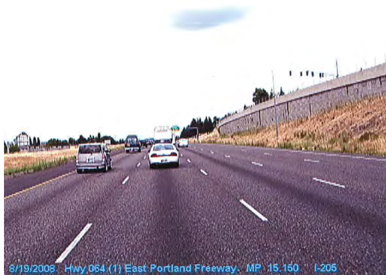
Figure 3.1: I-205 MP 15.15 showing pavement in good condition.
