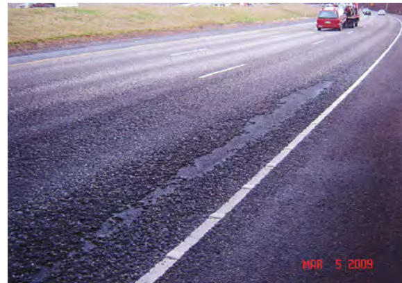
Figure 3.3: Pronounced raveling on I-205.
