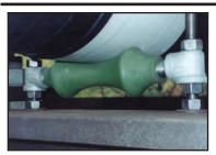
**Prevent the passing** of current from the pipeline to bridge structure, rebars, etc.
